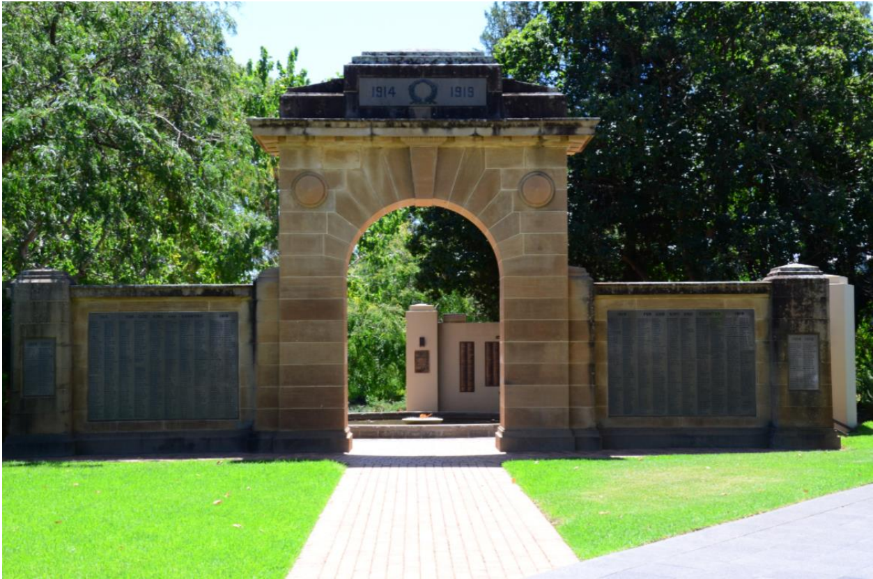
Wagga Wagga War Victory Memorial Arch (Photos from AWM – Places of Pride – Henry Moulds)
